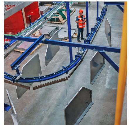
Installation of SLO 50 conveyor.
